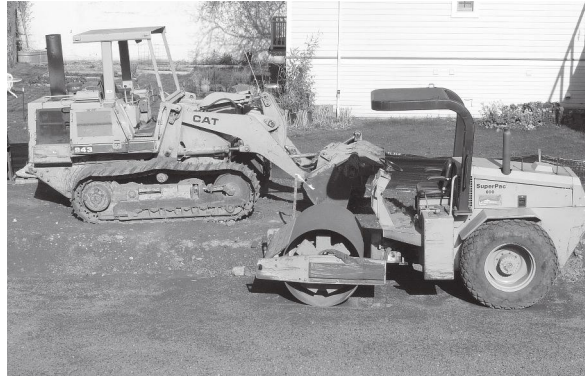
Front end loader and compacter.
