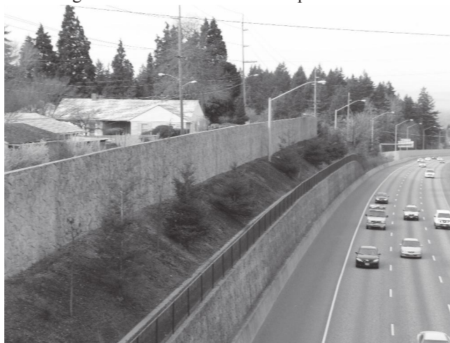
Rubber on asphalt means noise, which causes diminished property values and requires noise mitigation such as sound walls.
