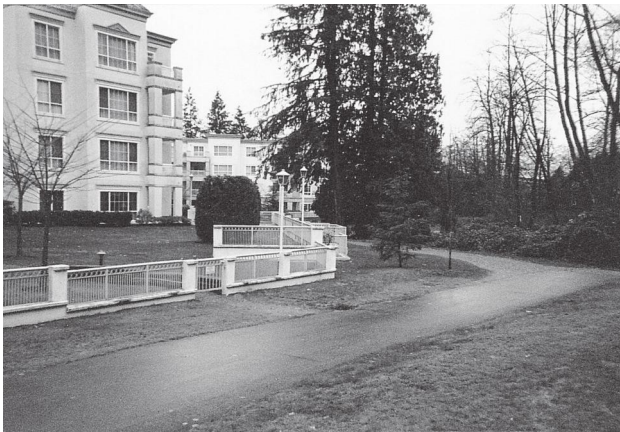
A paved path between an apartment complex and open space.
