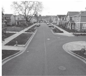
Residential street - paved, with curbs, sidewalks, and planter strips
