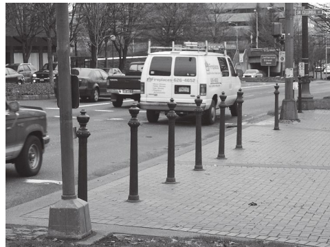
Removable posts - pedestrians and bicycles can pass with ease, but not vehicles
