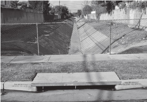
Concrete lined storm ditch
