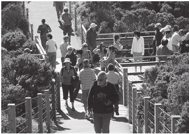
Fencing used to keep people out of sensitive areas.
