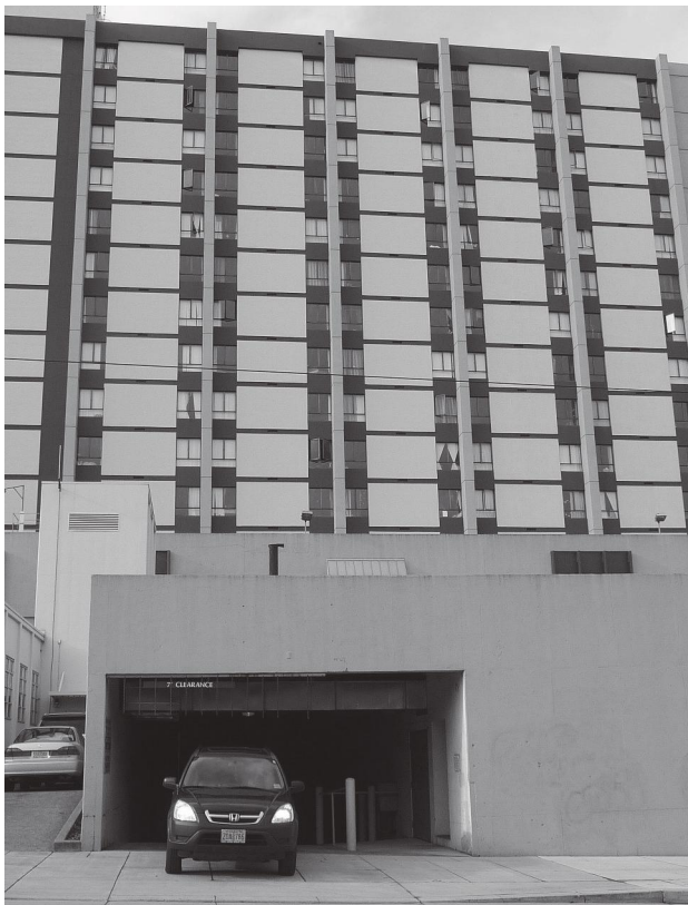
This apartment building has underground parking - literally, a buried cost passed on from developer to building owner to tenants.
