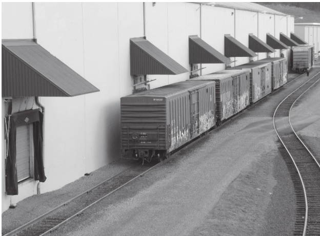
Railroad spur track accessing a factory or warehouse.
