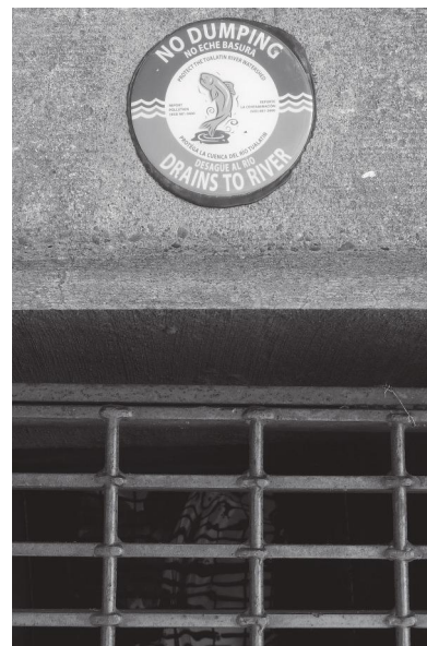
Inlet leading directly to streams and rivers.
