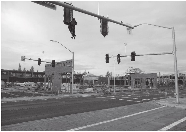
Construction of a new commercial development - Its generation of traffic creates the need for new traffic signals (in this particular case, the need for three new signalized intersections).
