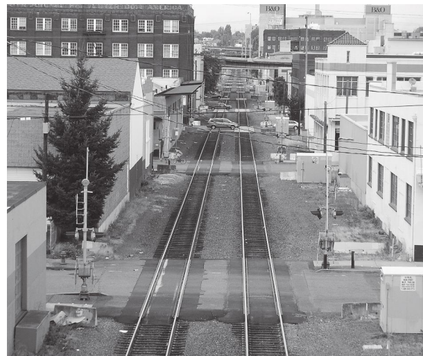
20 meter railroad right of way through an industrial district.
