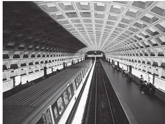
Below ground subway and station.
