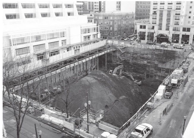
New downtown construction.
