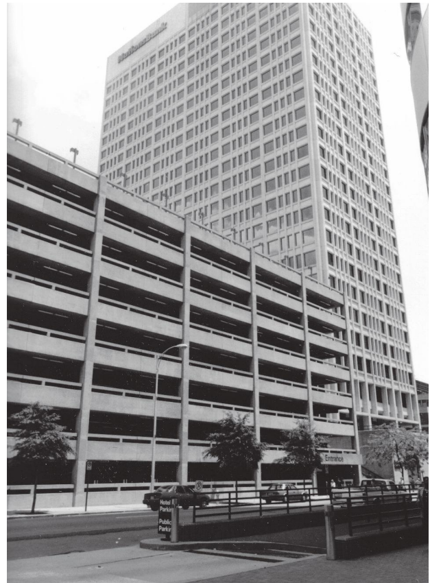
An office building and its accompanying parking structure. The parking structure's volume nearly matches that of the office building it serves.
