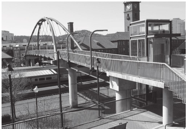
A pedestrian foot bridge crossing over railroad tracks.
