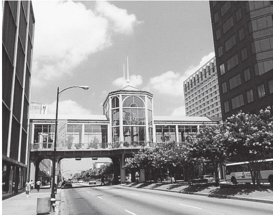
Skybridge - a good way to join buildings for a safer way to cross busy streets and especially nice in cold or wet climates
