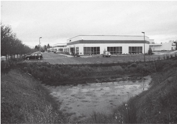
Parking lot detention pond designed to filter out oils and grime. It is a future Hazardous Material Site in the making.
