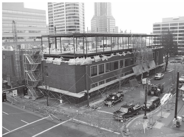
Consideration for future upward expansion of buildings is an integral part of Pedestria's building code and minimum height requirements. Here another floor is being added to an existing 2 story building.
