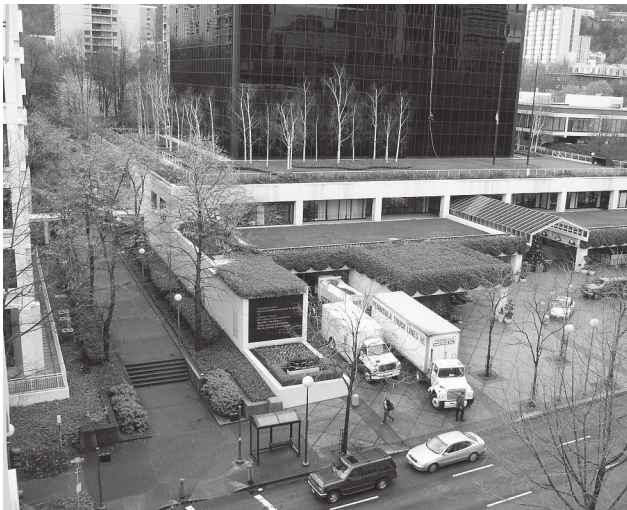
Office building - freight loading dock.
