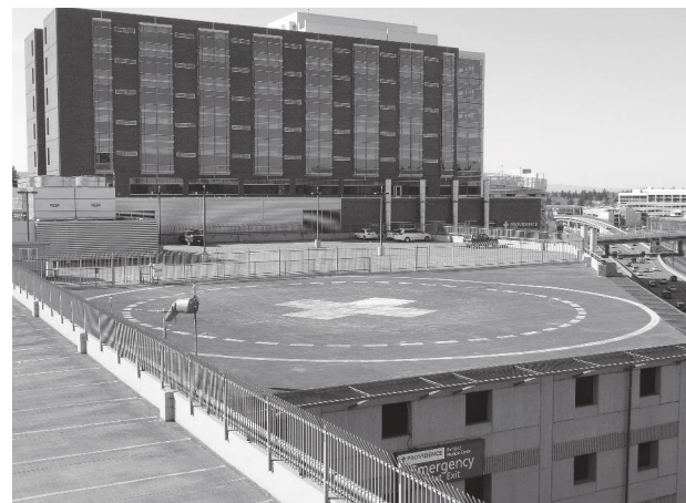
Helicopter landing pad on top of a hospital complex
