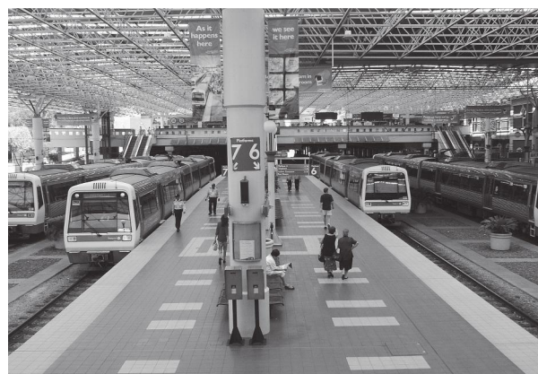
Transit loading platform - Pedestria's is very similar, except for a serrated edge and buses rather than rail trains.
