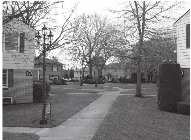
2 story apartment buildings
