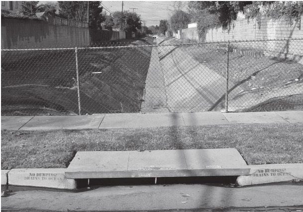
Concrete lined storm ditch
