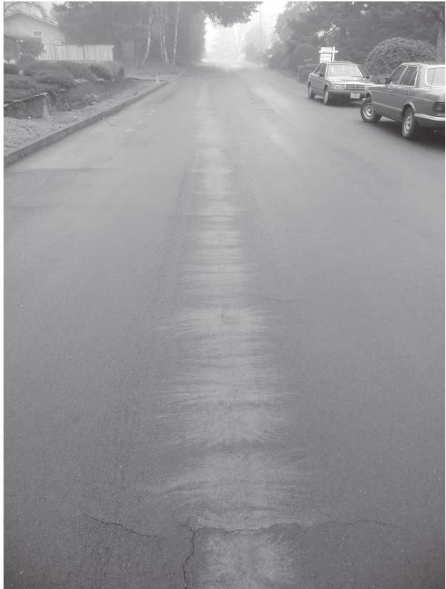
Someone's car leaked oil all the way down the street.
