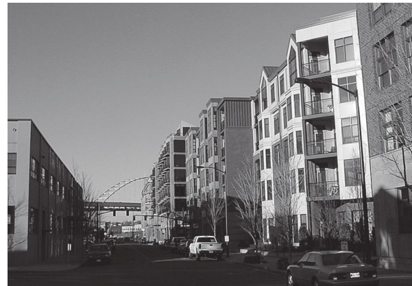
Medium rise residential buildings
