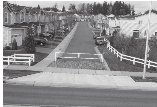
Gate - opened only for emergency vehicles and for special permitted occasions.
