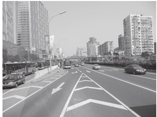
For safe and functional roads and highways, striping is a necessity. It is often repainted every year.
