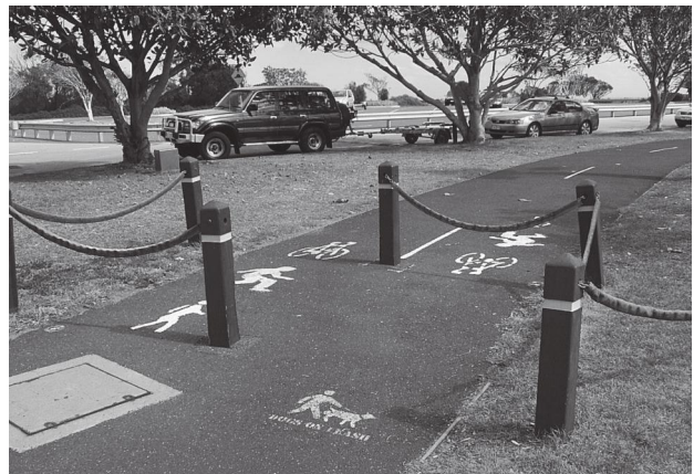
There may also be places where physical barriers are necessary to slow bicycle traffic down.
