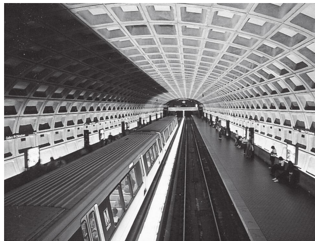
Below ground subway and station.
