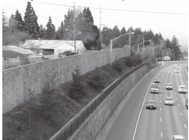
Rubber on asphalt means noise, which causes diminished property values and requires noise mitigation such as sound walls.
