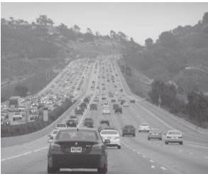
Major urban freeway - no pedestrians or bicycles allowed.
